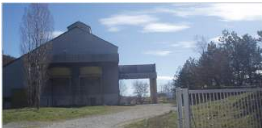
Figure 3-97: Silo de stockage GPS – Mirabeau
