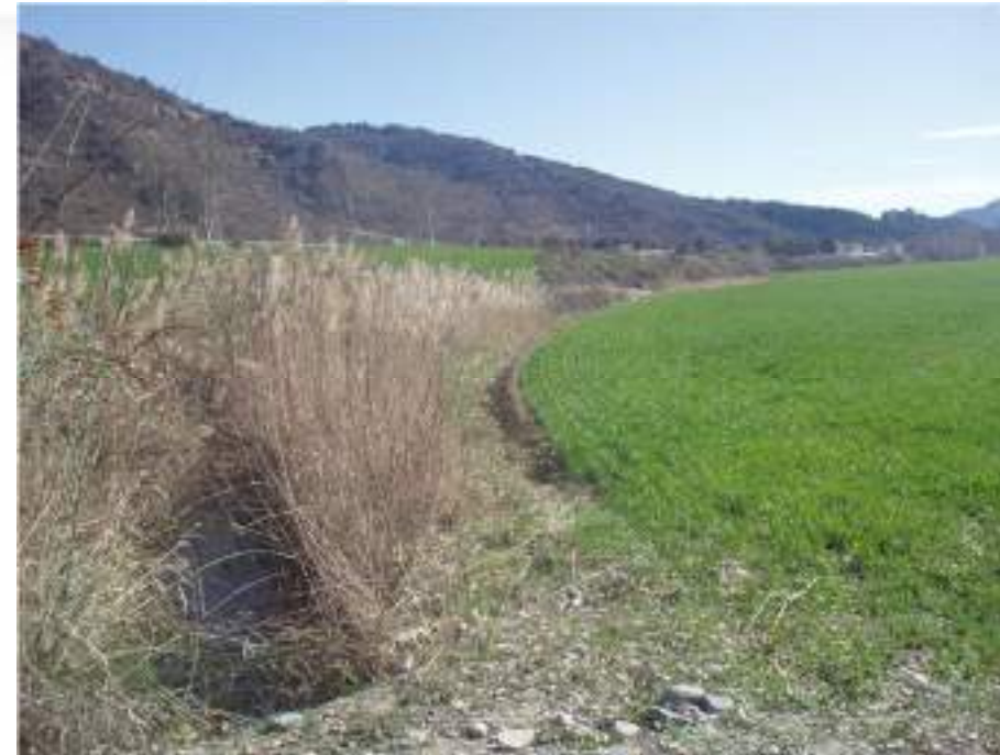
Figure 3-89: Canal gravitaire – Mirabeau
